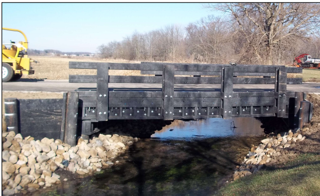
Bridge 174-0.56 over the Onion Ditch
